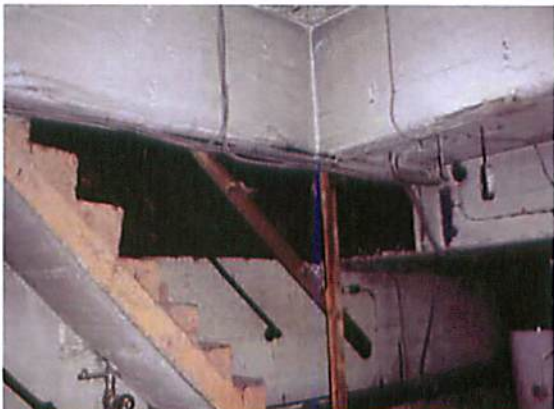
Fig 4.1.13 Original theatre basement
