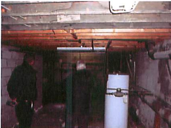
Fig 4.1.12 Original theatre basement
