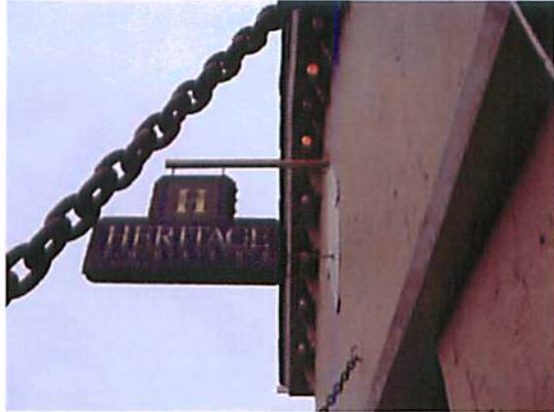
Fig 4.1.2 View of signage on west elevation
