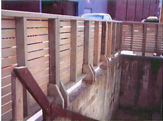
Fig 4.1.7 Stairs down to dressing room basement
