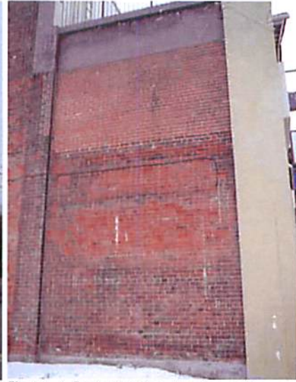
Fig 4.1.6 East elevation showing early rear addition and 2005 exterior improvements.
