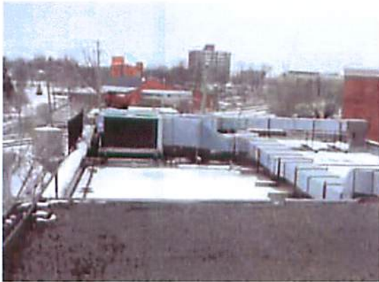
Fig 4.1.9 Roof looking east
