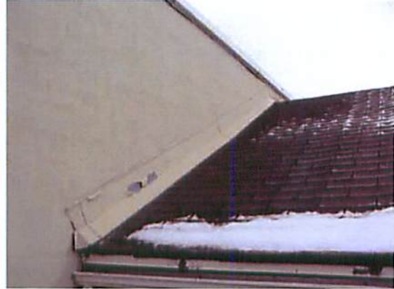
Fig 4.1.8 View of pitched roof on west elevation
