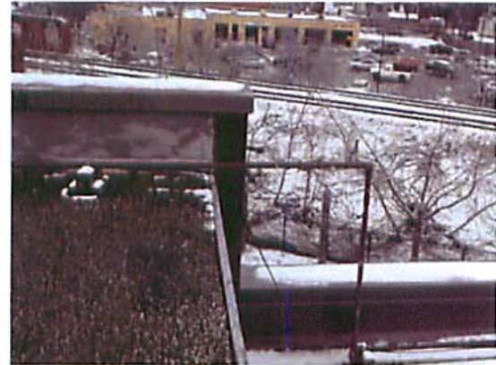
Fig 4.1.10 Roof showing step down from balcony level to main assembly area
